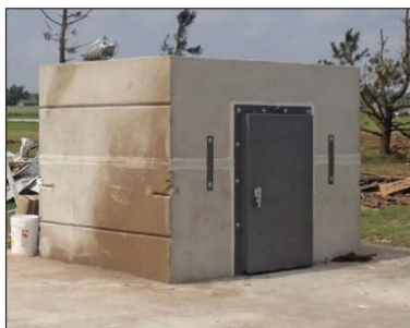
Stand-alone room near a house still intact after a tornado (FEMA Taking shelter from the storm, 2014.)
