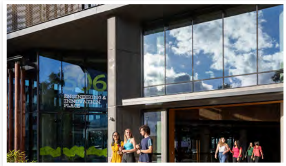
Engineering and Innovation Place, JCU Townsville, Bebegu Yumba campus, Douglas
